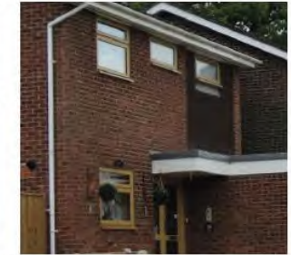
Timber framed windows and doorway.
