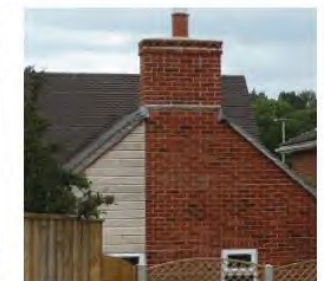
Wood weatherboarding adjacent to red brick facade aligned to chimney.
