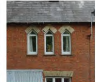
Brick lintel detailing above fenestration.
