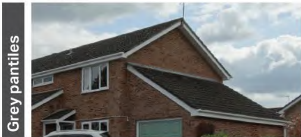
Gable roof with skillion roof attachments over the garage and entryways.
