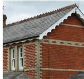
Brick detailing along the window line and corner. Decorative fascia pattern.
