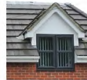
Gable dormer with painted timber casement window.
