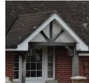
Timber frame gable dormer porch with render filling.
