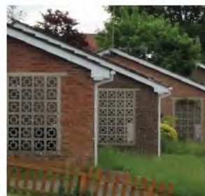
Decorative concrete panes in brick porch wall.
