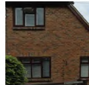
Dark wood frame casement windows.
