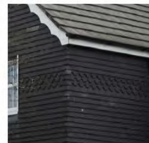
Continuous pattern in weatherboards and decorative fascias.
