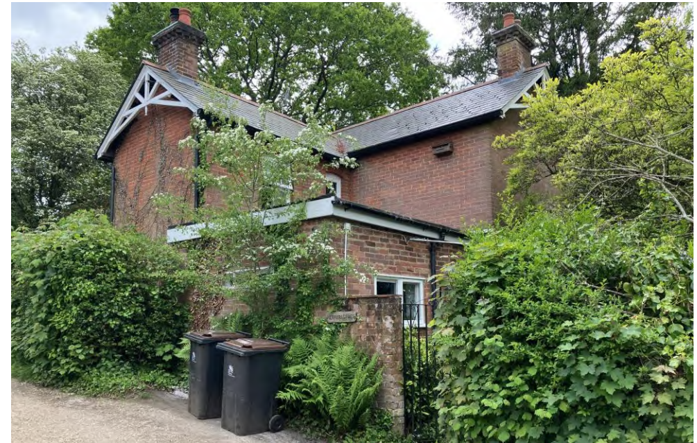
Figure 13. Decorative gable end, ridge tiles and chimneys
